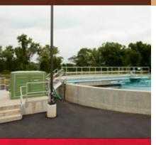
This ReliaSource® Above-Ground Submersible Valve Package (ASVP) utilizing SF Series® solids-handling submersible pumps transfers sludge at a wastewater treatment plant.
