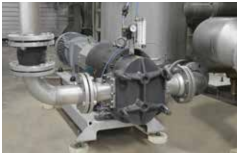
ONIXline pump for conveying Starch Slurry
