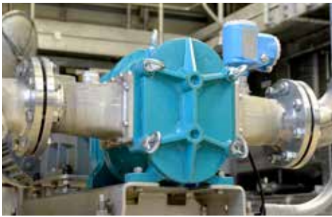
BLUeline pump for conveying cleaning agents.
