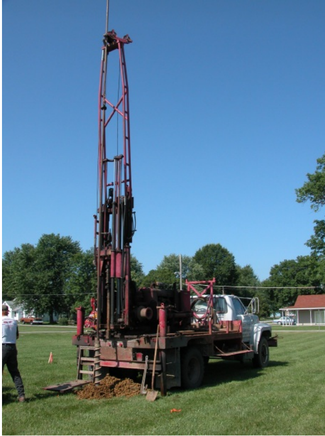
Auger Drilling Operation Figure 2-7
