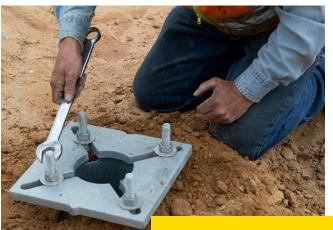
Variable bolt circle styles allow for fast bolt-up as the slotted design mates with most light standards.
