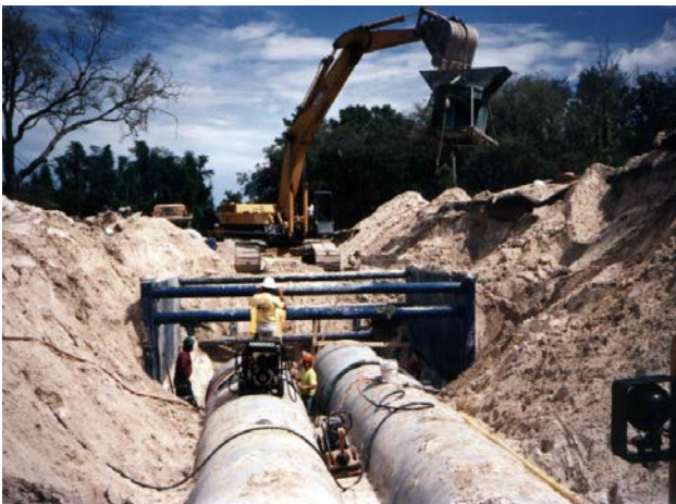
On this job the Hydra-Tech S3TC, 3" dewatering pump was used to keep groundwater under control on this pipe laying project.
