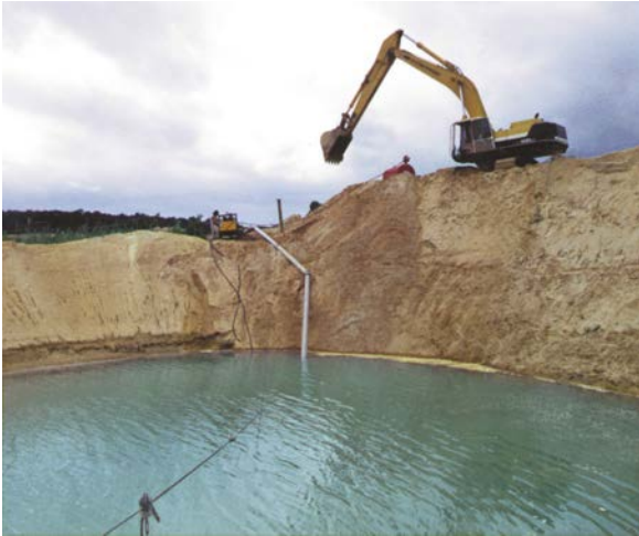
6" submersible pump driven by the HT60DCV diesel power unit was used to divert ground water at a sand plant
