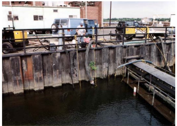
This job required divers, using Hydra-Tech's S4THLDI pumps fitted with suction hoses, to remove silt deposits in a power plant intake flume.
