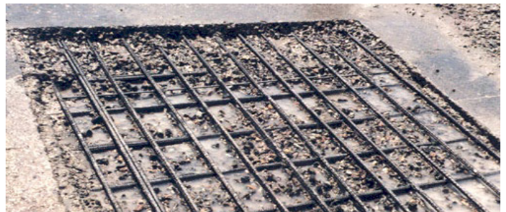
Descales & cleans rebar without damaging the reinforcing grid.
